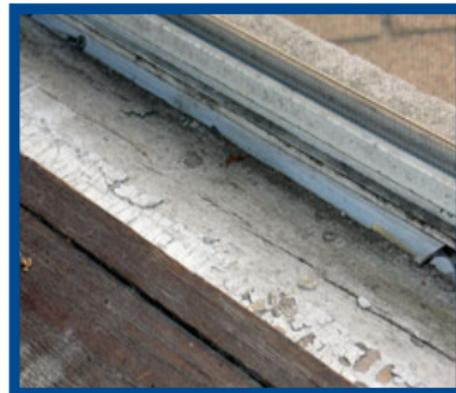
When old paint cracks and peels it creates **lead dust**, too small to see with the naked eye. Windowsills are a common place to have lead dust.
